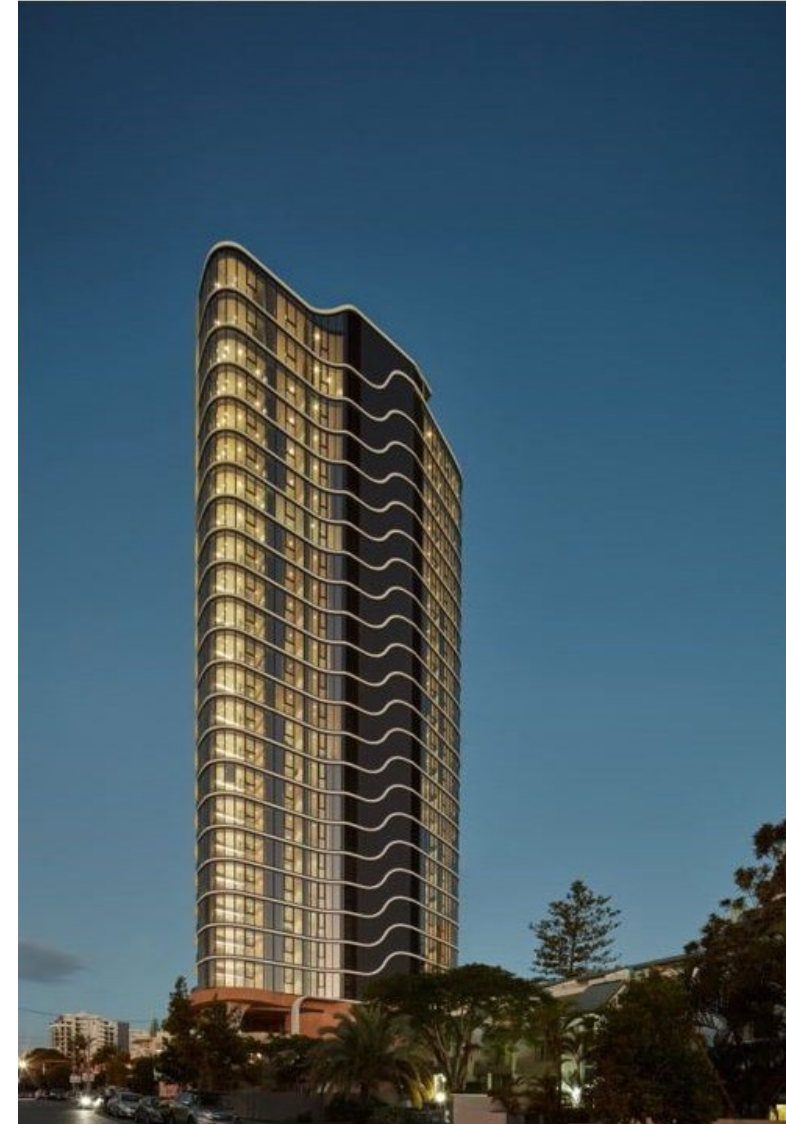
Encore, Broadbeach (Andrews Projects)
